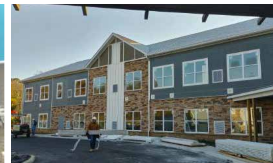
Harmony at Anderson (under construction)
