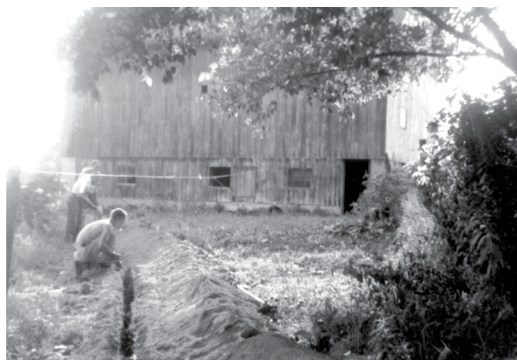
Digging a trench off the barn, date unknown.
