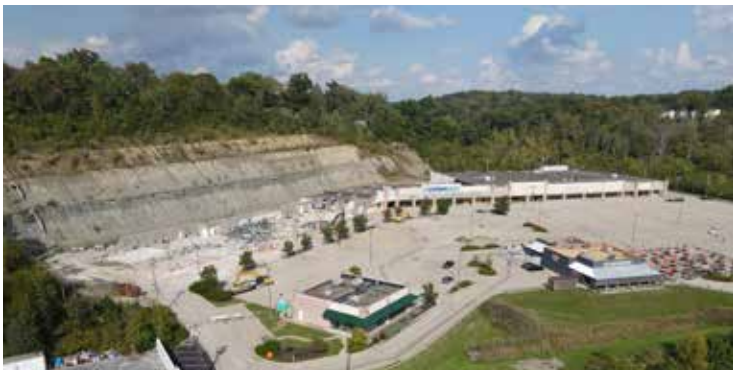
Demolition at Skytop Pavilion was completed in October.
